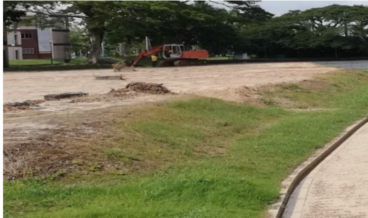
Figure 1. Construction Site at Curtin University Sarawak
