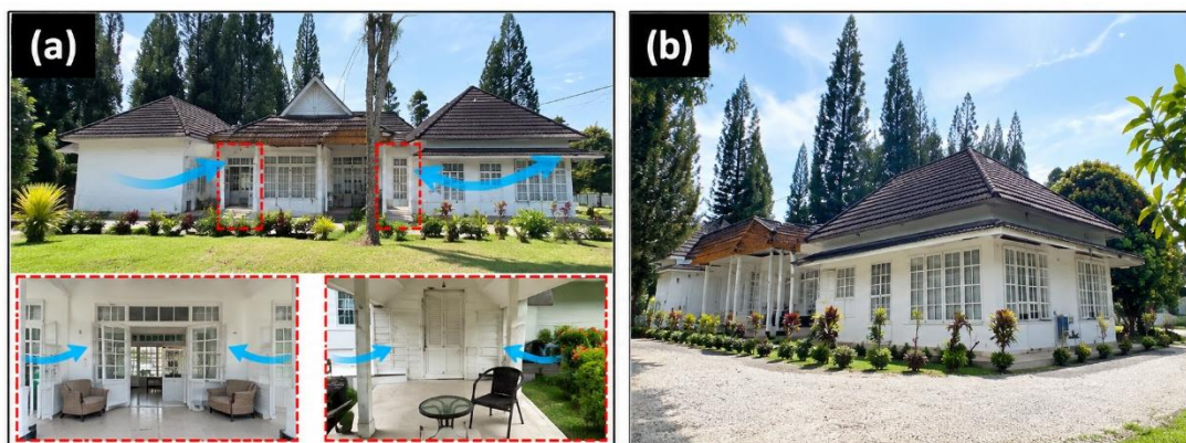
Figure 3. Cross-ventilation through the arrangement of façade openings (a); side vegetation surrounding the building and providing natural shading (b).
