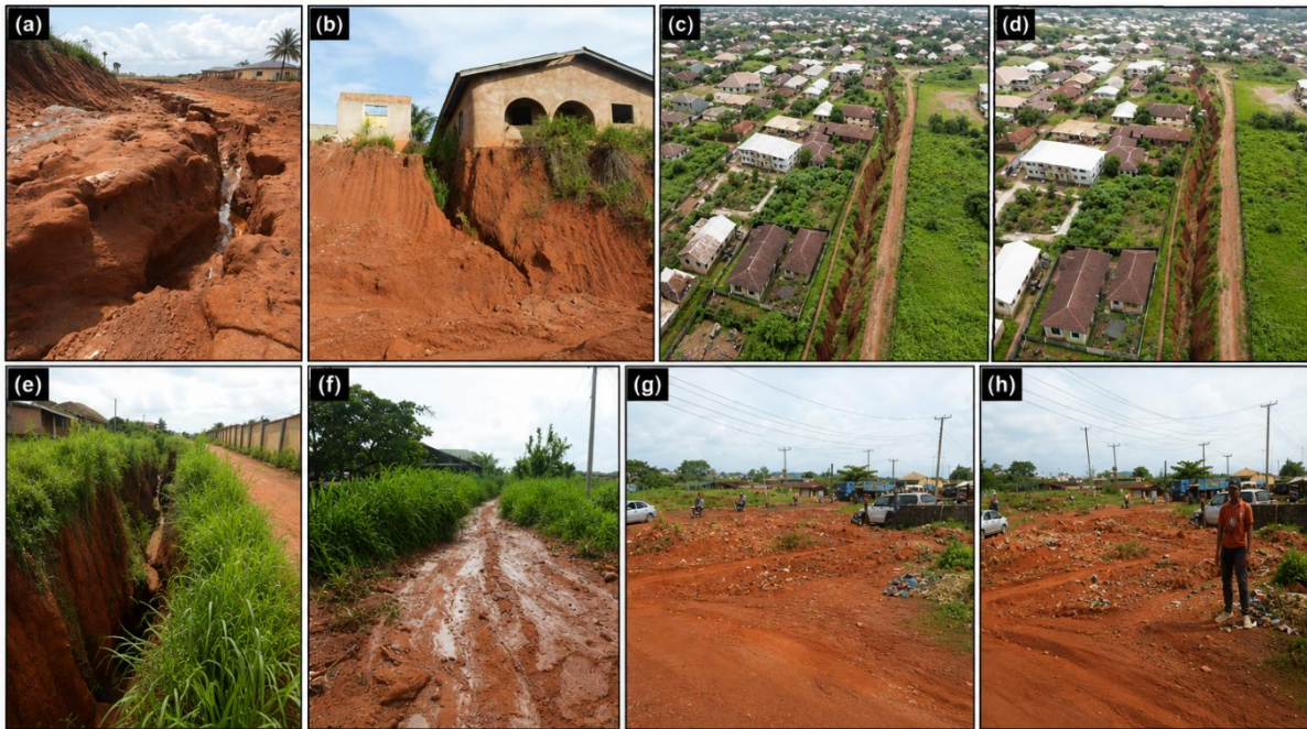
Figure 3. Erosion gullies in Agbor metropolis: (a) rill-to-gully development at Midoma; (b) abandoned houses along the Midoma/Iweriebor erosion wadi; (c–d) aerial views of the Alibuba erosion wadi; (e) affected houses along the gully perimeter; (f) downstream section of the Alibuba wadi; (g) sand deposits across F222 (F109); and (h) soil and waste deposits along F222 (F109).
